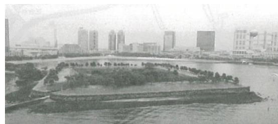
Current state of the third battery
