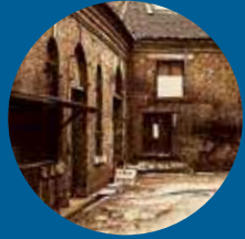
官営品川硝子製造所 (1960年代中頃) Government-operated Shinagawa Glass Factory (mid 1960s)
