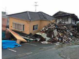
A building collapsed due to earthquake shaking (the 2016 Kumamoto earthquakes)
