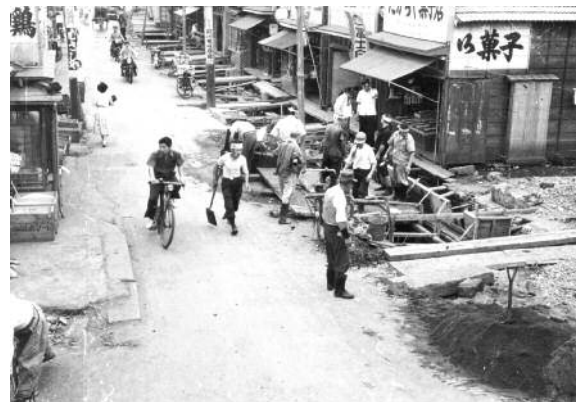
▲ Construction to cover the Shinagawa Irrigation Canal (1954)
