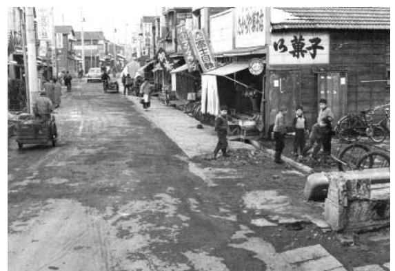
▲ The same street after construction finished (1954)
